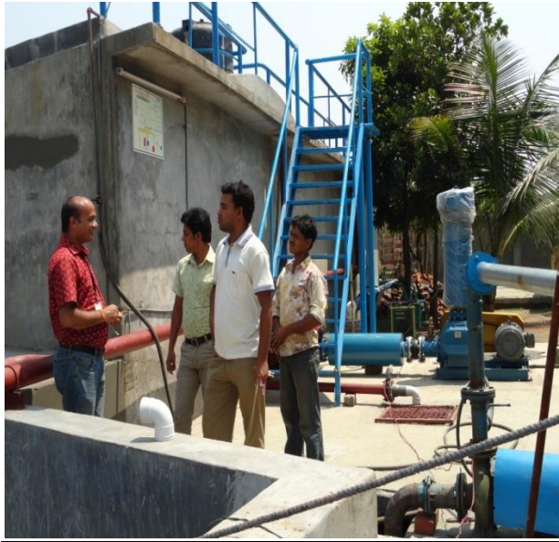
Air Blower Installation
